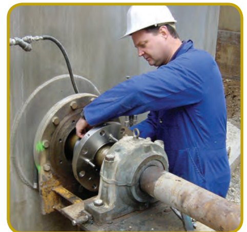
INSTALLING THE 4.5 IN. FULLY SPLIT EA TYPE-1 SEAL ON BLACK LIQUOR AGITATOR
