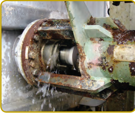
BEFORE: STUFFING BOX ON A 4 IN. PAPER STOCK AGITATOR.
