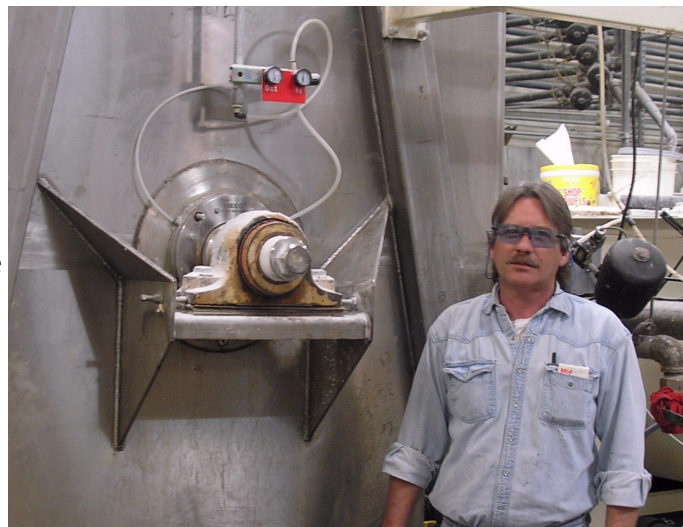
Plant technician Chuck Dowdy stands beside the blender with the MECO seal mounted and purge lines connected.
